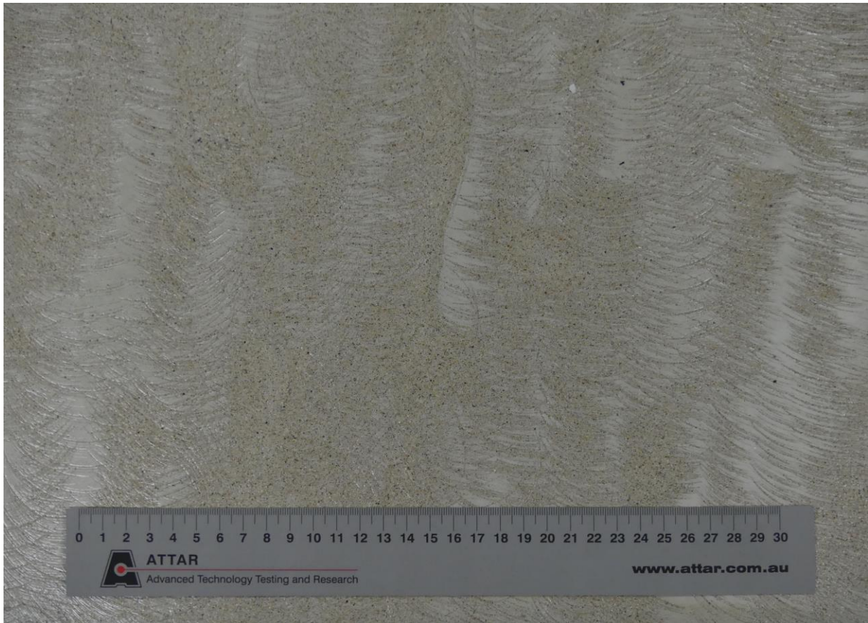
Figure 1: Dulux Avista 2 Pack Urethane Sealer applied to steel trowel finish concrete
