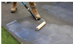
Apply Dulux Avista Sealed Surface Primer OR Bare Concrete Primer per application instructions.
