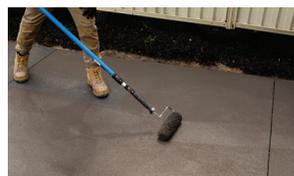
Apply Dulux Avista Waterbased Tintable Base Concrete Sealer per application instructions, allowing it to dry in between coats.
