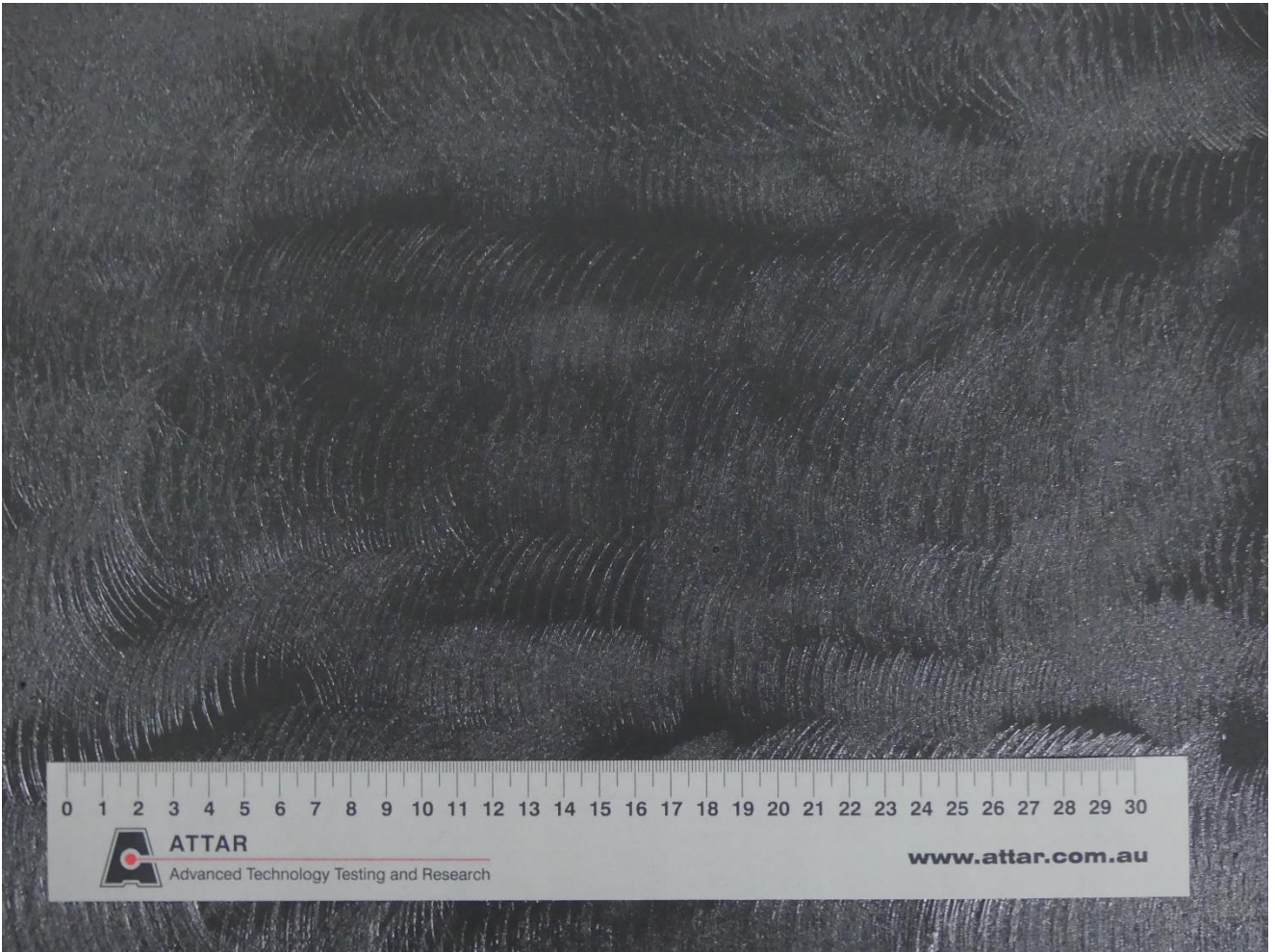
Figure 1: Dulux Avista Tintable Base Sealer applied to steel trowel finish concrete.
